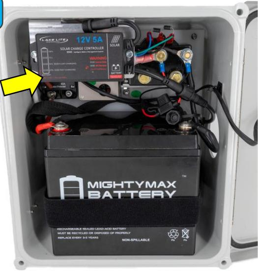
Secure the solar charge regulator anywhere inside the box
